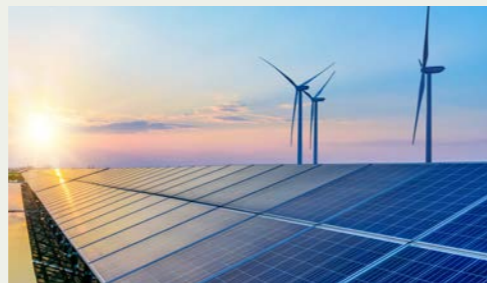
Solar panels contribute significantly to reducing our plants' carbon footprint. We installed more than 6,000 solar panels on the roof of our Avelgem plant , generating 3,076 MWh per year.
