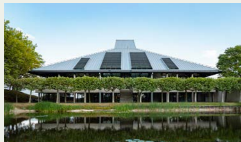
The IVC Flooring Development Centre in Waregem (Belgium) has been turned into a sustainable base. It uses heat recovery, intelligent lighting technology and is powered by solar panels on the building.
